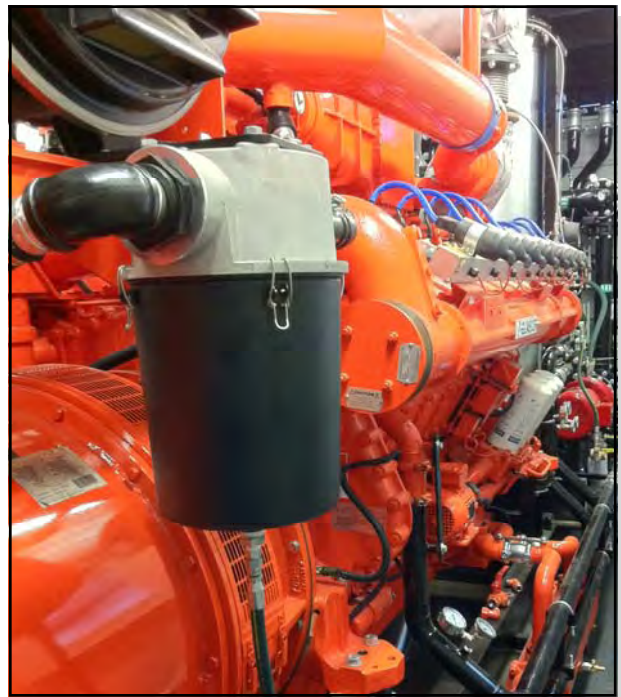
Closed Crankcase Ventilation System Guascor Engine Installation
